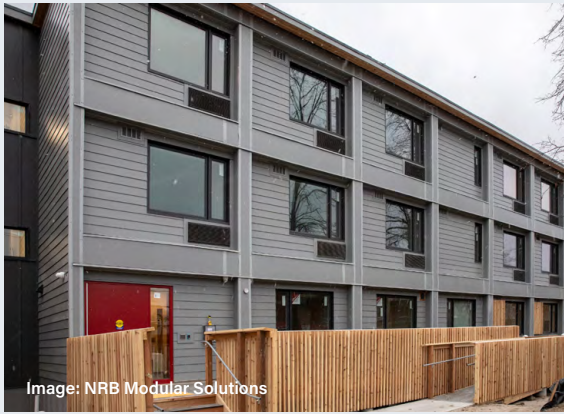
Built by NRB Modular, constructed using volumetric modular method, this building provides 100 affordable single-occupancy rental suites in Toronto, Ontario [2].
