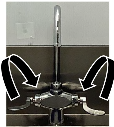
Figure 23: Wrist blade orientation of the splash study faucet (left), where the faucet is turned on by rotating the wrist blades upward, and a faucet with standard wrist blade orientation (right), which is turned on by rotating the wrist blades left or right.
