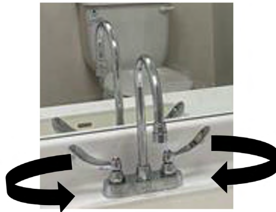
Figure 23: Wrist blade orientation of the splash study faucet (left), where the faucet is turned on by rotating the wrist blades upward, and a faucet with standard wrist blade orientation (right), which is turned on by rotating the wrist blades left or right.
