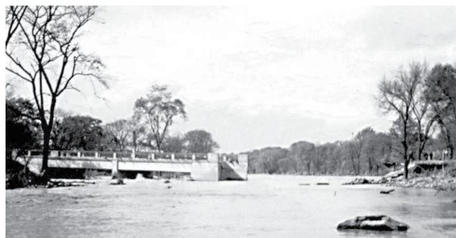
Figure 5: Bridge damage due to Hurricane Hazel, 1954. Source: Martin Taylor, https://creativecommons.org/licenses/by-sa/3.0/deed.en
