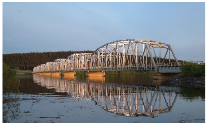
Figure 20: Nisutlin Bay Bridge, Yukon Territory. Reproduced with permission from Associated Engineering.
